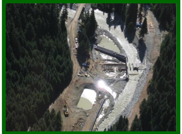
Fitzsimmons Creek Hydroelectric Power Project intake – construction phase.
