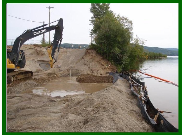
An excavator removes contaminated soils from the ground near Watson Lake, Watson Lake Airport, YT.
